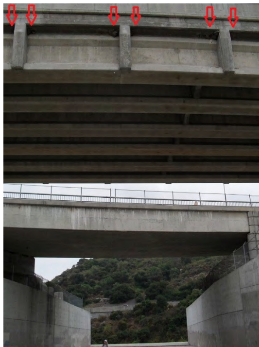
Photo 2: Facing south depicting north side of the Spillway Crest with active cliff swallow nests under the overhang on each side of the support beams.
